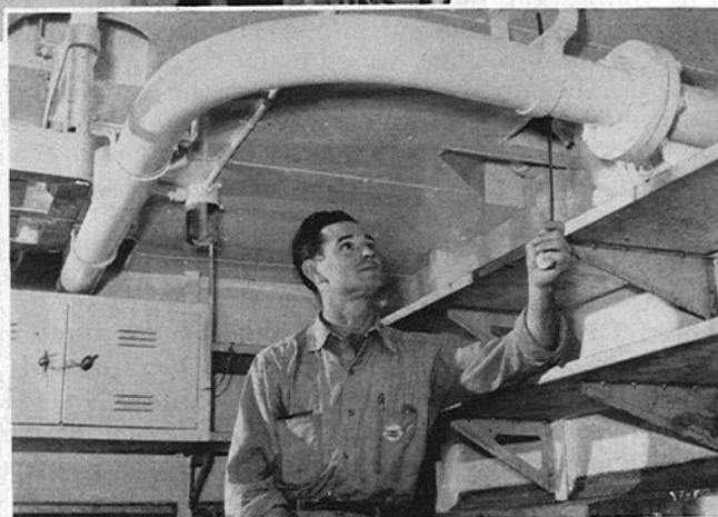
This plumbing drain is typical of the intricate work done on installation. The scene is the galley.
