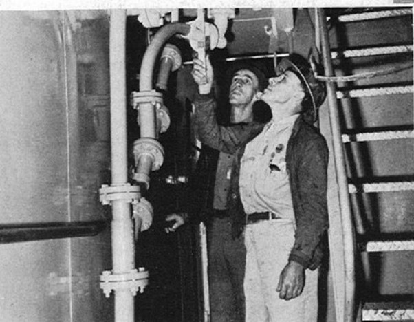
Here is "the Christmas tree" as the drain piping forward of the galley is known. A real tricky installation.
